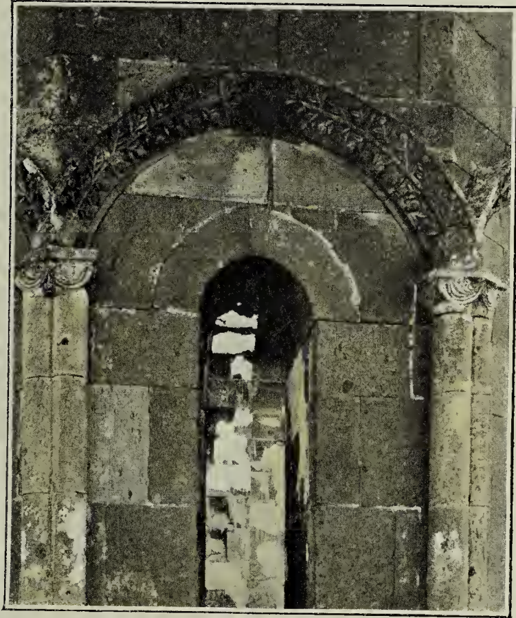
FIG. 63. MOULDINGS ON NORTH SIDE OF RUINOUS CHURCH AT TALIN.
